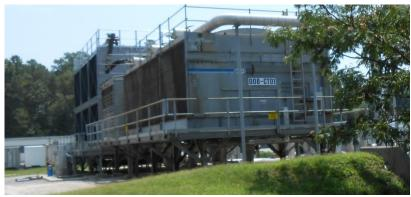
Scope: The existing CHL #1 cooling tower is at the end of it's useful life. Existing cooling towers serving process cooling loads at the CHL Buildings will be demolished and replaced with two (2) larger cooling tower cells to match the existing 12 GeV Cooling Towers recently installed during the 6MSD.
